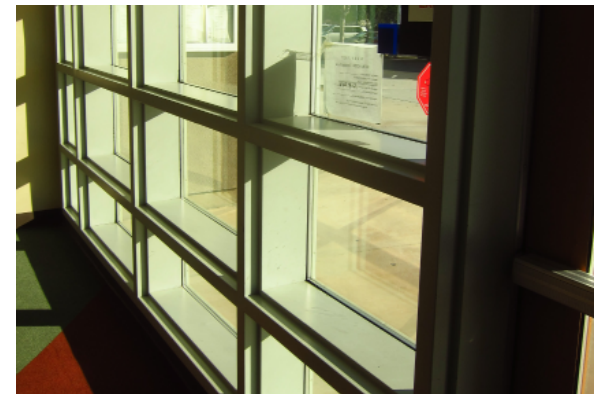
Typical exterior window condition.
