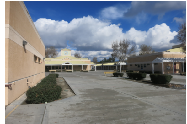
Exterior plaza and typical concrete.
