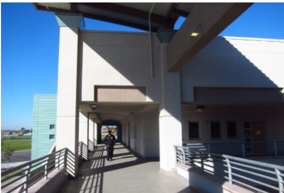
Second floor exterior walkway.
