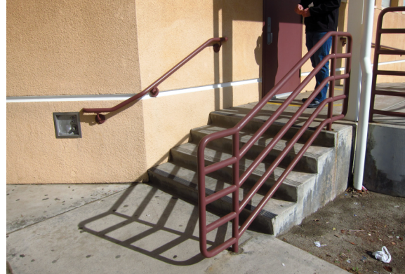
Stairs and railings to locker room office.
