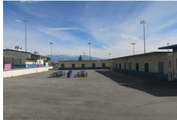
Hard courts/ Main Quad area; view towards portables.
