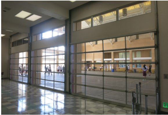
Glass sectional rolling doors between MPR and Gymnasium.
