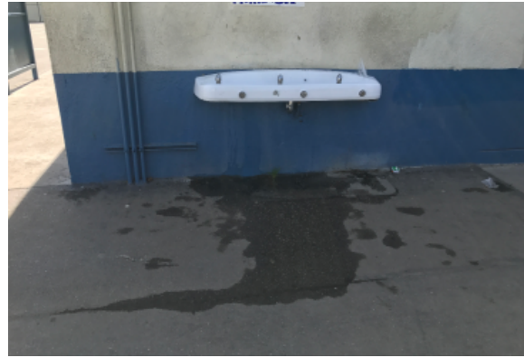
Typical drinking fountain.
