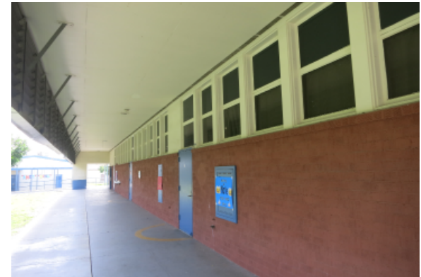
Typical classroom building.
