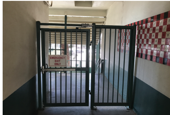
Typical tube steel fence and gate.
