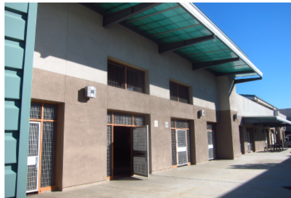
Typical building exterior.
