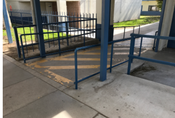
Ramp connecting main spine walkway to classroom wings.
