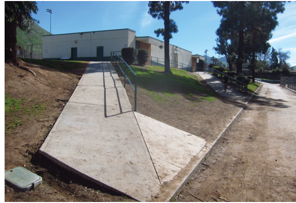
Inaccessible path of travel to locker room building.
