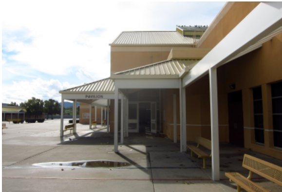
Typical building exterior and walkway.
