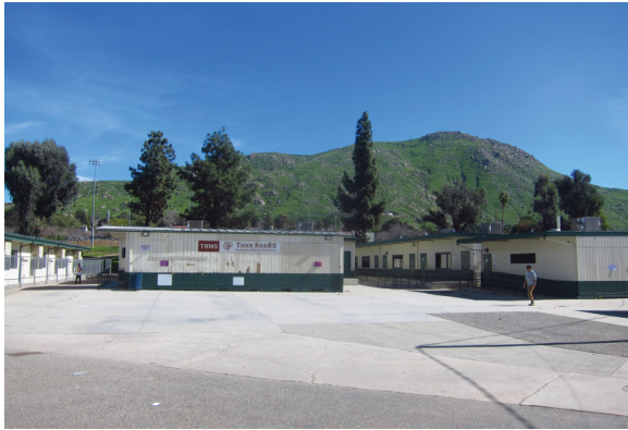
Significant quantities of modular classrooms across the site.
