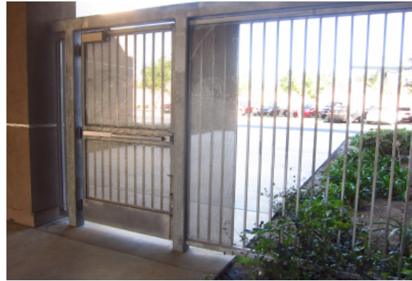
Tube steel fencing.
