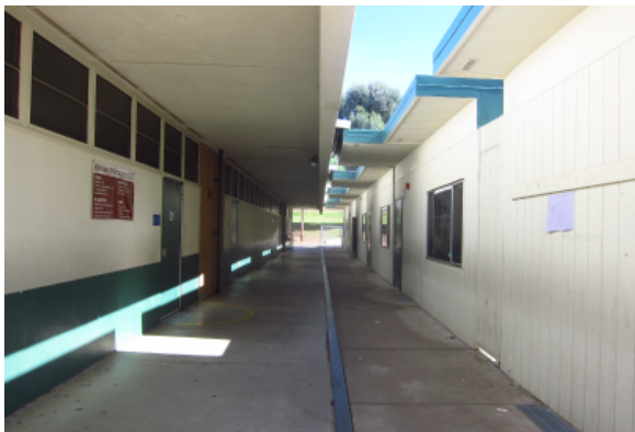
Typical exterior of permanent classroom building on the left and modular building on the right.
