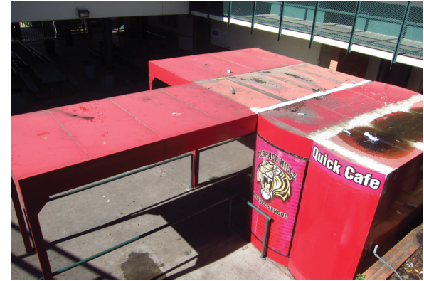
Quick Cafe food service satellite at outdoor dining sunken court.
