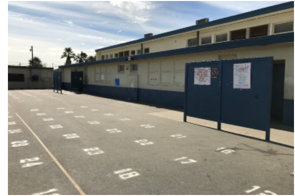
Locker room building.
