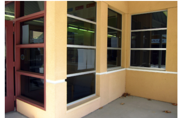
Typical exterior window condition.
