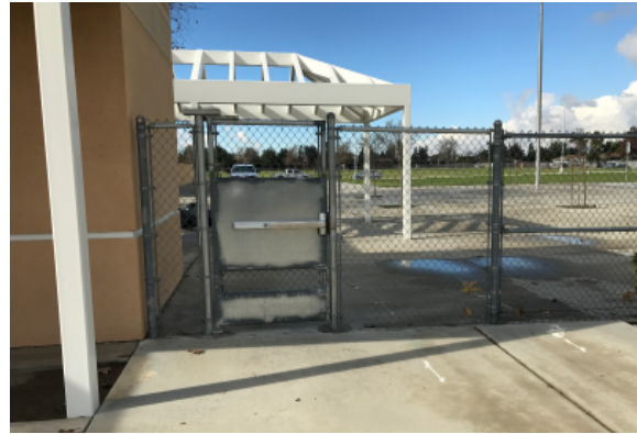
Chainlink fencing and gate.
