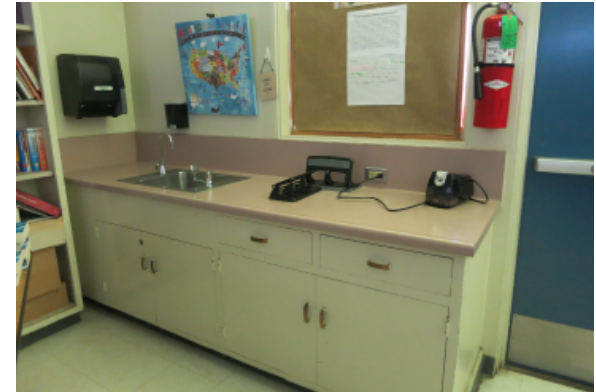
Typical classroom casework and sink.
