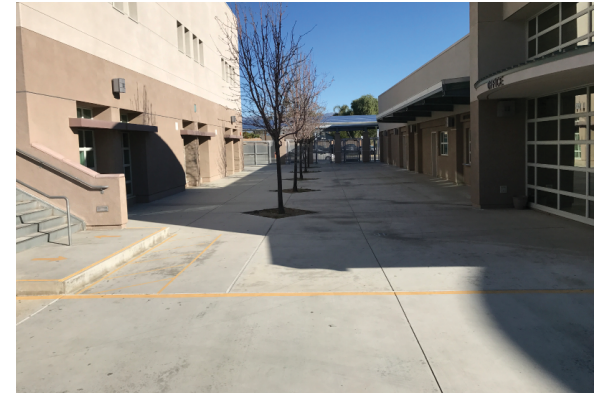
Typical exterior paving.
