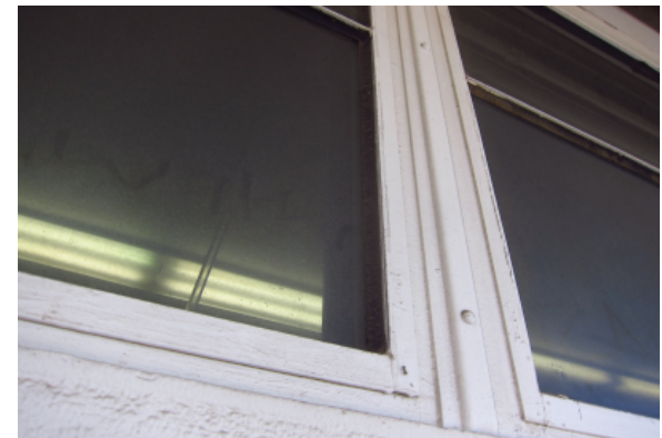
Typical exterior window condition.
