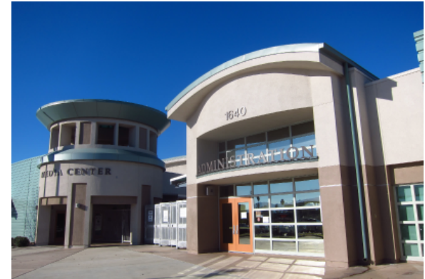
Front entry, Administration building, and media center.
