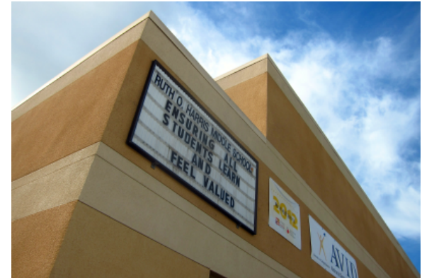
Typical building exterior plaster condition.
